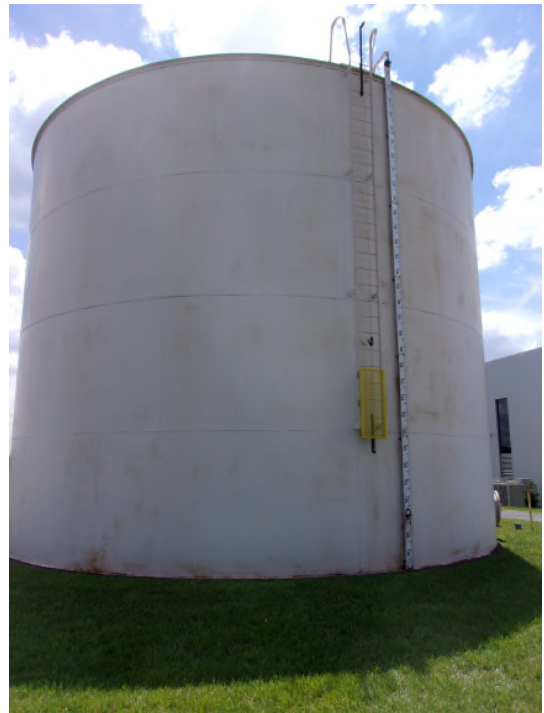
Photo #: 2 Description: Exterior Shell (4 Courses): Coating film degrading and exhibiting sporadic rust areas, Lower Shell course and circumferential chime shows the most severe corrosion areas.
