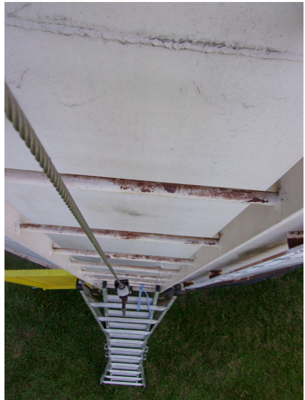
Photo #: 6 Description: Exterior Shell: Downward view of ladder rungs and shell.
