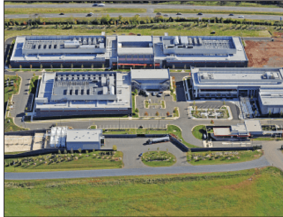
Figure 2-6 Source: Equinix: CU3 Culpeper Data Center
