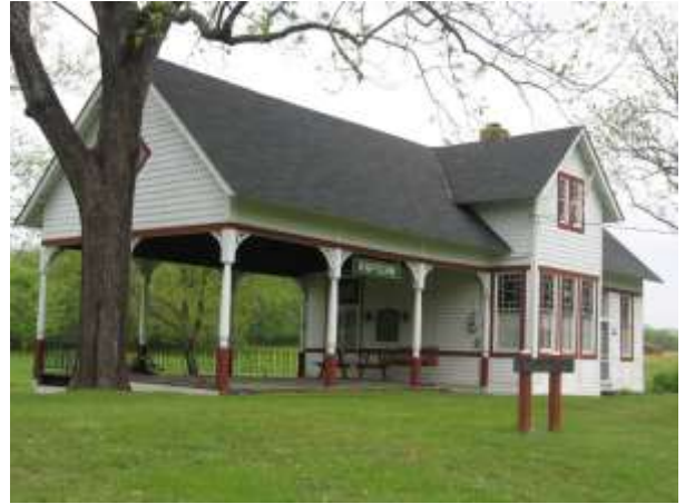
Rapidan Passenger Depot, Photo by Dovetail Cultural Resources Group
