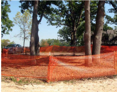
Tree Protection: Safety Fence installed around the drip line of trees to protect the root system
