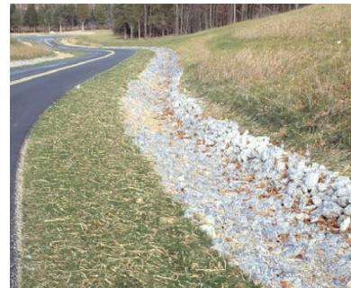
Stormwater Conveyance Channel: Channels can be grass, rip-rap, or concrete. Used to convey water away from property
