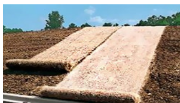
Stabilization Blanket: Should be installed per manufactures recommendation
