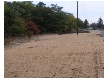
Seeding & Mulching: Seed/Straw should be applied within 7 days after final grade is achieved
