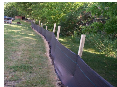
Silt Fence: Stakes should be at least 5' long and spaced no more than 6' apart
