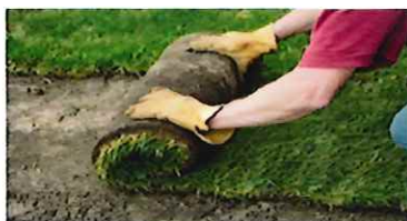
Sodding: Sod should be laid in staggered rows and installed within 36 hours of being cut
