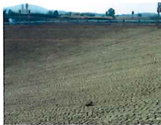
Surface Roughening: Slopes should be tracked so grooves are oriented horizontally
