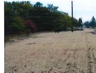
Seeding & Mulching: Seed/ Straw should be applied within 7 days after final grade is achieved
