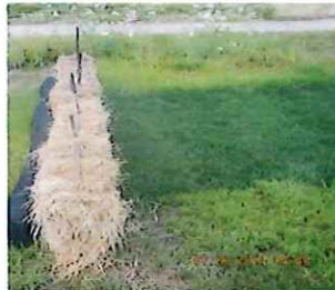
Straw Bale Barrier: Two Stakes per Bale with bale entrenched and backfilled
