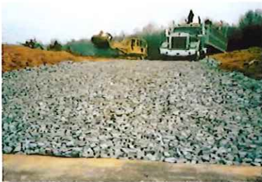
Stone Construction Entrance: VDOT # 1 Stone with Filter Fabric Underlayment
