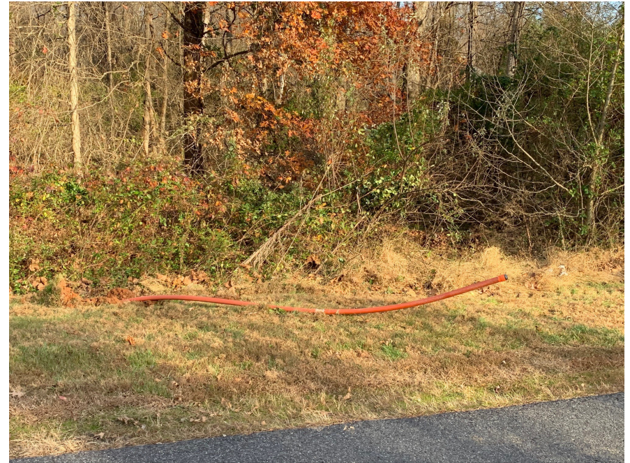
On the roadside—Fiber being installed
