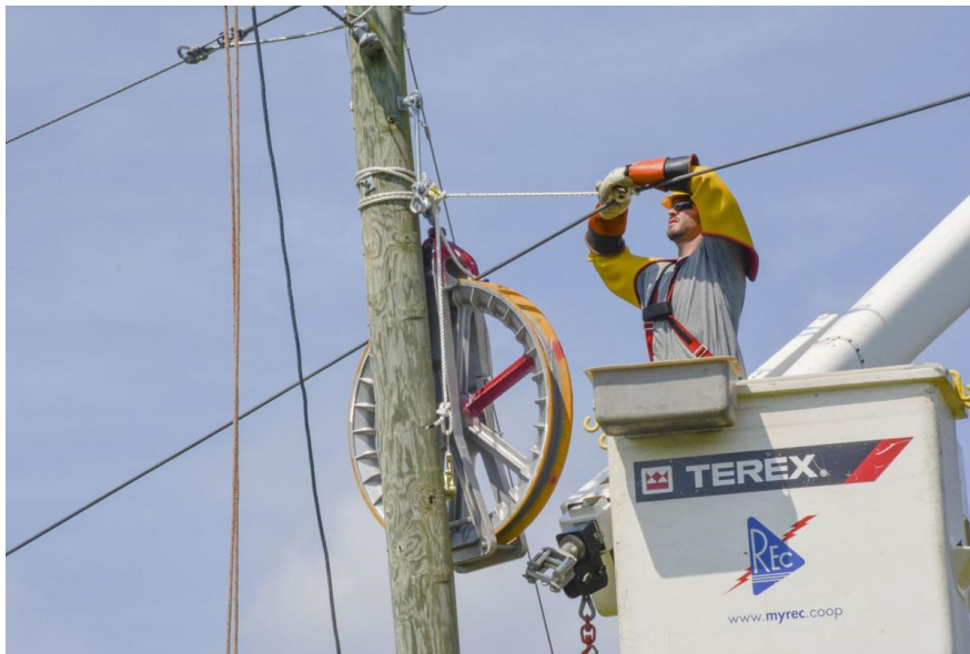
A lineman tends transmission hardware on REC's network. RAPPAHANNOCK ELECTRIC COOPERATIVE
