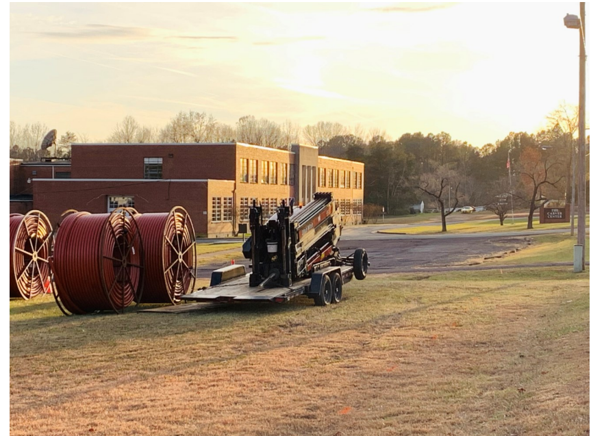
Fiber Optic cable rollout to the Carver Center on State Route 15
