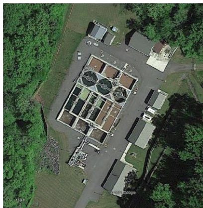
Arial View of Culpeper County Sewer Plant at Clevengers Village.
