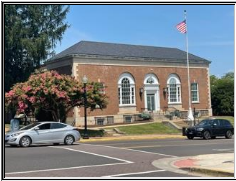
Culpeper County Administration Building
