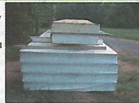
SIP's waiting to be raised
