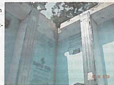
Inside corner of foundation
