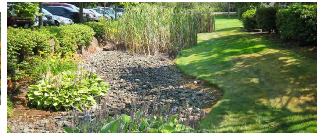
Bioswales integrated into a landscape, filtering and retaining water from the adjacent parking lot.
