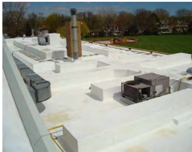
Cool roofs reflect the sun's energy back into the sky instead of the energy being absorbed into the building.
