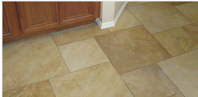
Porcelain tile is highly durable, and most tiles have potential to contain recycled or regional materials.
