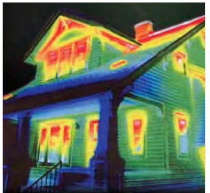
Green is good. Blue is better. Infrared images show locations (red, yellow and orange) where heat is escaping.
