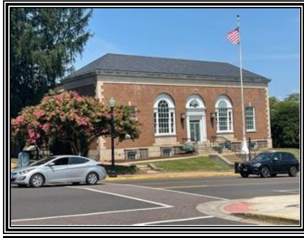
Culpeper County Administration Building
